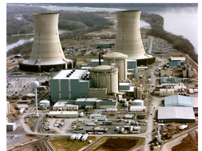
Figure 15.21: Three Mile Island nuclear plant in Pennsylvania. The two reactor cores are in the foreground of the larger cooling towers behind. Source: U.S. DoE.
