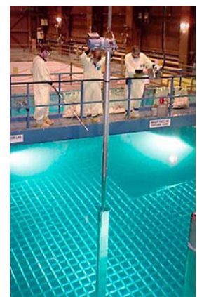
Figure 15.20: A spent fuel rod being lowered into a storage grid in a pool of water at a nuclear power plant. Source: U.S. DoE.
